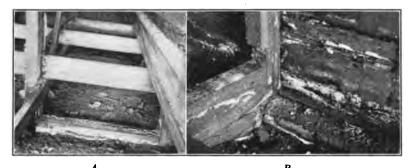
Fig. 39.—Spread of fungus by contact. A, open shed where infection has spread upward from decayed piece on ground. B, corner of building where infection has spread from decayed sill.
